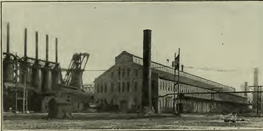
FIG. 1. GENERAL VIEW NORTH END OF GARY WORKS, NOS. 11 AND 12 FURNACES, WITH NO. 3 BLOWING HOUSE
